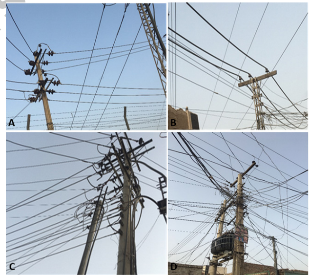
Fig. 3. Suspended wire on 11kV Tata Pur Feeder (A), 1000MCM cable is used in 11kV line (B), Dangerous Pole (11kV) (C) and Dangerous Pole (400V) (D).
