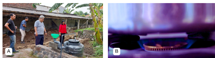
Figure 3: (A) Installation of the biogas digester 550 L at the dairy cattle farm in Bendul Merisi Village. (B) The biogas was channeled to the stove and produced a blue flame.
